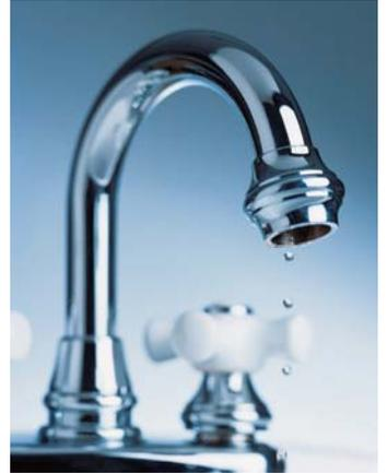
If your faucet leaks around the handle only when the water is turned on, you need to replace the packing - the pliable material beneath the hexagonal nut. Coat the threads of the stem with petroleum jelly and reassemble the faucet.
